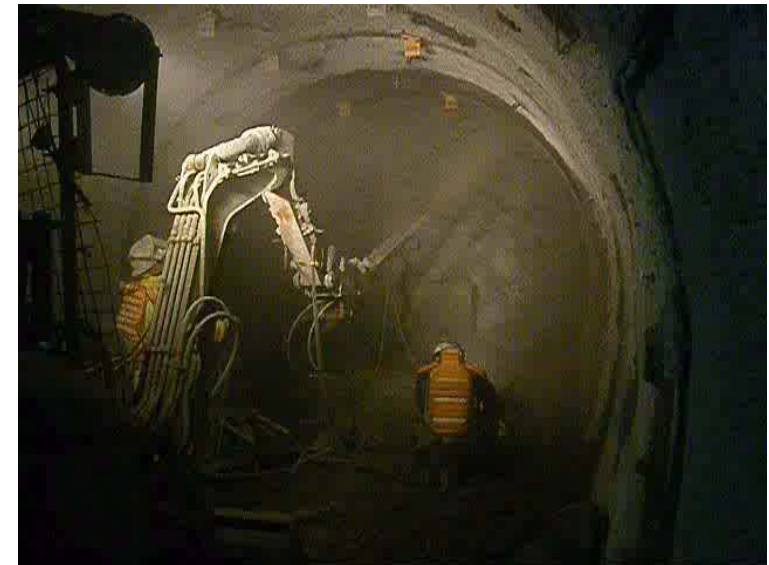
In-situ shotcrete demonstration test at Horonobe URL: July, 2009
